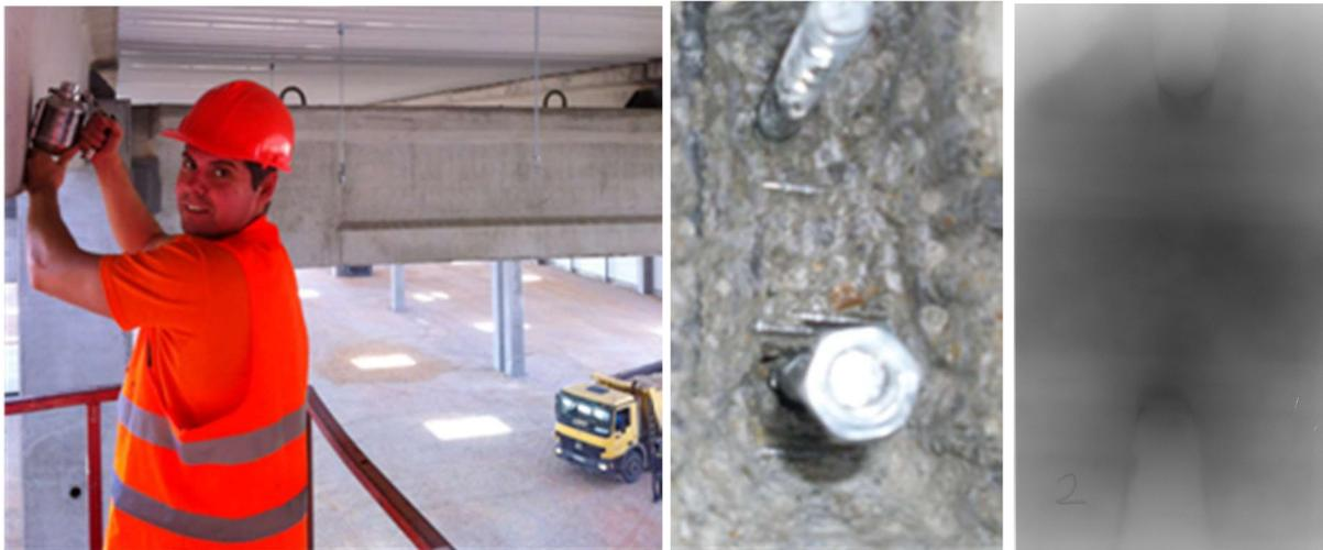
**Fig. 3.29 and 3.30 Moment of carrying out control, detail and radiographic images of anchors bolts and tensioning ropes in the connection "steel column – reinforced girders"**
