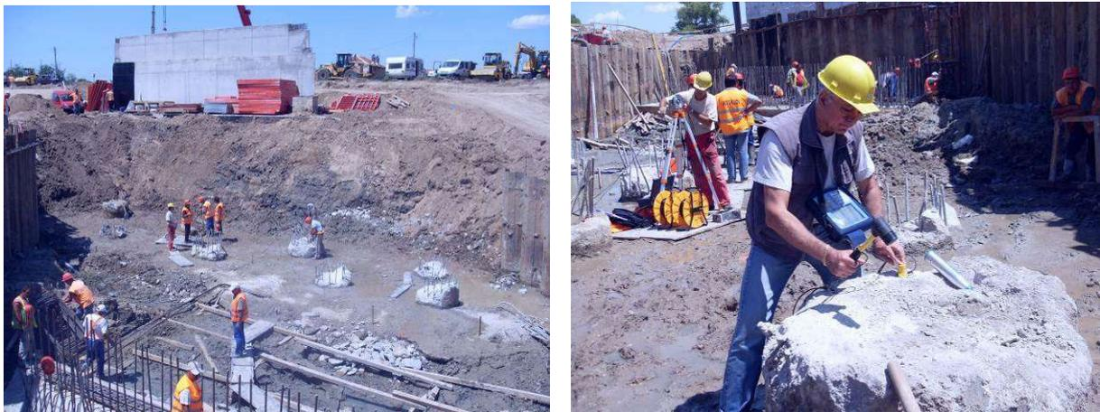
**Fig. 3.33 and 3.34 General view of the executed piles of pole P1 and a moment of the combined test of the integrity of their two methods – a "TDR 2" and "Ultrasonic Cross hole Testing" (in the background)**
